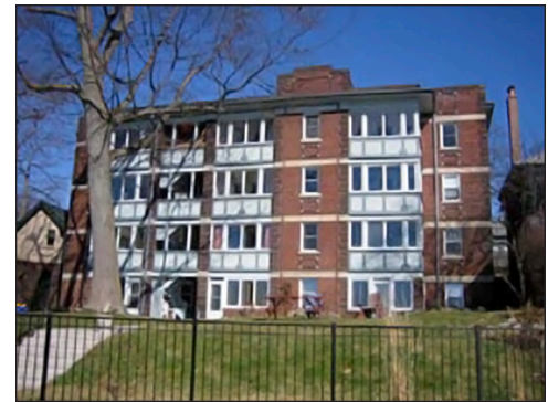
This photo taken before the original Tudor panels were replaced shows the (now capped) scuppers at the lower edge of each verandah/sunroom.
