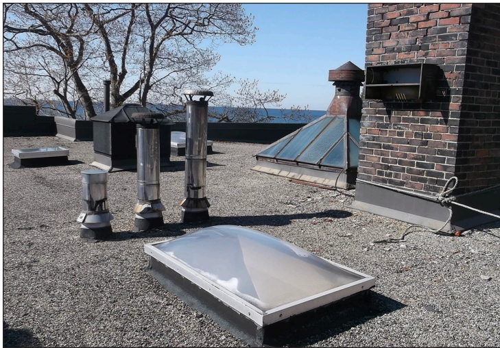
The original skylight with its cupola top. The three metal stacks are for the newer wood-burning fireplaces, and the shorter capped chimney in the background tops the ventilation shaft for the stack of bathrooms without windows. The metal box on the side of the chimney might be either part of an early lightning rod or the housing for an electric retrofit of the cupola fan.
